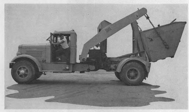
THE DEMPSTER DUMPSTER hoists one of the away. Here Charlie A. Monroe, 4215, checks to see huge trash buckets spotted throughout the area onto that the big bucket is being hoisted properly. its back and trundles off to dump them five miles
